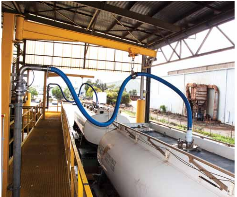
The new liquid loading system with two filling points on a dedicated weighbridge allows for simultaneous filling of both front and rear trailers. Liquid fertilizer load out has been reduced to as little as 20 minutes.
