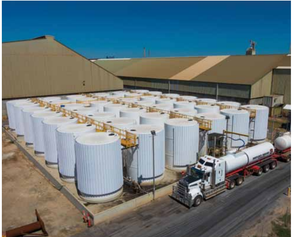
Summit has doubled the Kwinana liquid fertilizer storage capacity. Flexibility of despatch times and hours of operation is another cornerstone to the business.
